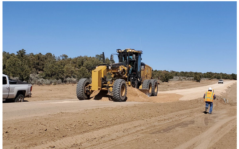
Limestone being spread on C-429 South.
