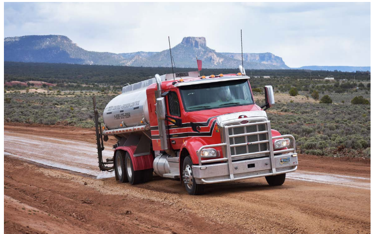
DuraBlend being applied to C-321.
