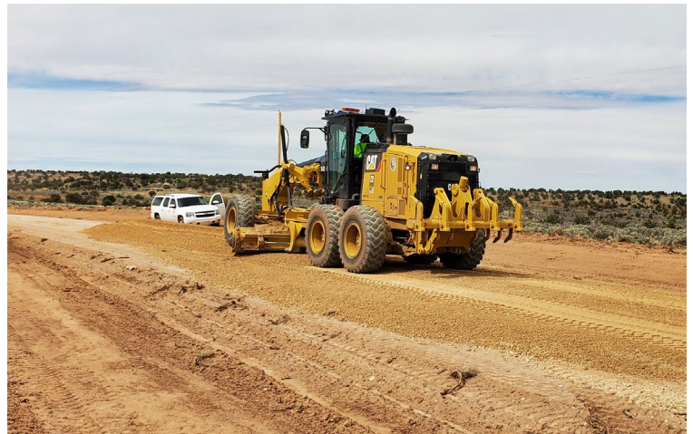
District 2's preparation work on C-321 project.
