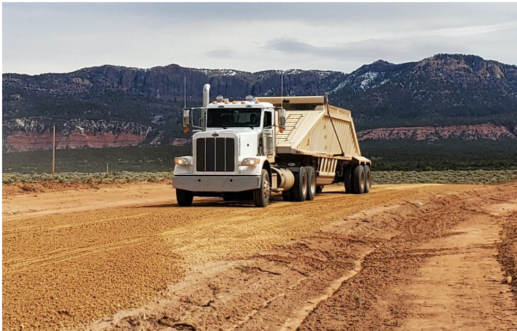
Limestone being hauled to C-321.
