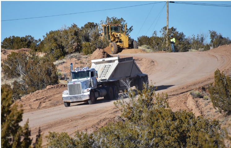
Limestone being dropped off on C-302.
