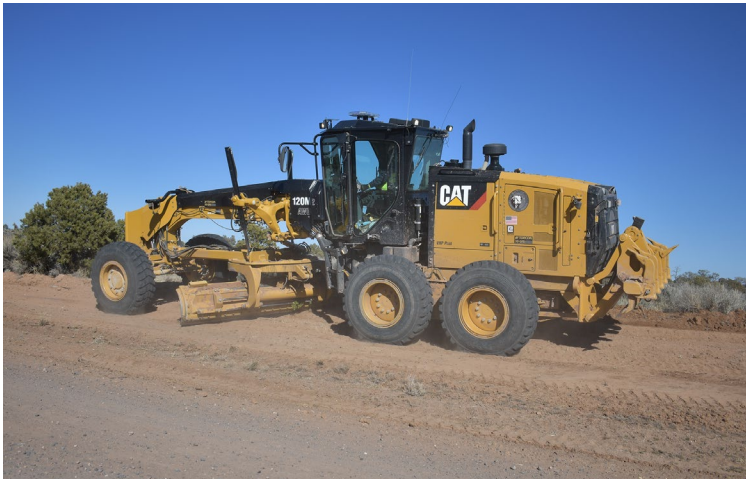
Road Maintenance continues.
