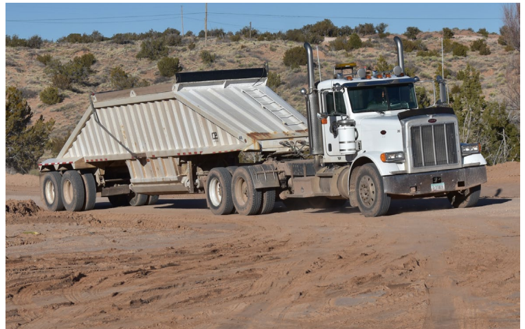
Continued limestone hauling.
