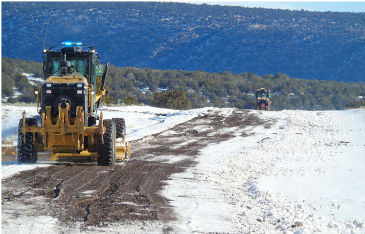
Graders blading county roads.
